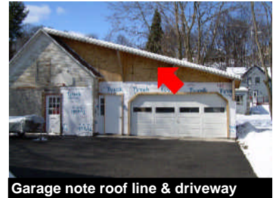
Garage note roof line & driveway
