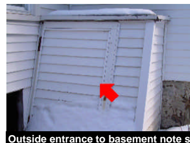
Outside entrance to basement note sr
